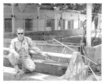
(Side) Typical wash stand. These are found throughout Afghanistan near bathrooms. Most bathrooms are pit toilets; these stands help improve health and hygiene. This one is fed from an elevated water tank supplied by a solar pump in a well. Most places in Afghanistan lack electricity so solar pumping is a reliable way to provide water.
